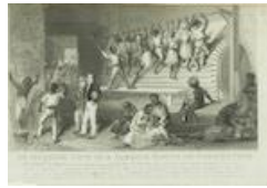
Figure 76. An Interior View of a Jamaica House of Corrections.
